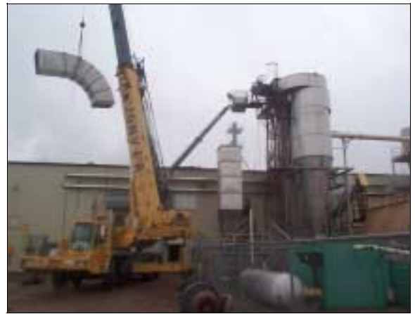
Installation of a corn dryer
