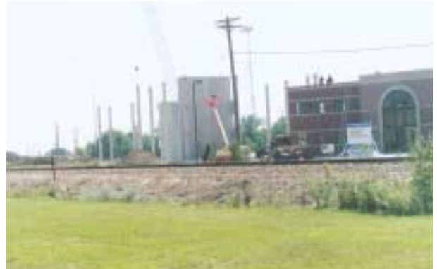
Construction of new complex that will house Pinnacle offices..
