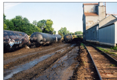
Tanker cars are moved out of the way as clean up operations get underway.
