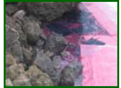
Pads were placed along the rocky River's edge to soak up the fuel.
